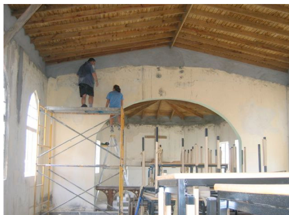
Mark and Marla Ree begin the interior reconstruction at St. Albans.
